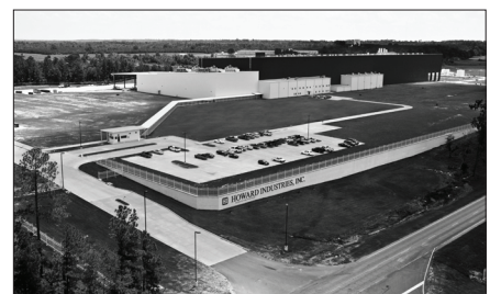
Figure 2: Howard Industries Substation Plant, Ellisville, MS
